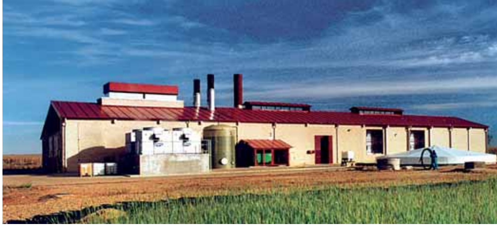
OTSI S.A. power generation plant San Millán with two V16 TCG 2032 series engines.
